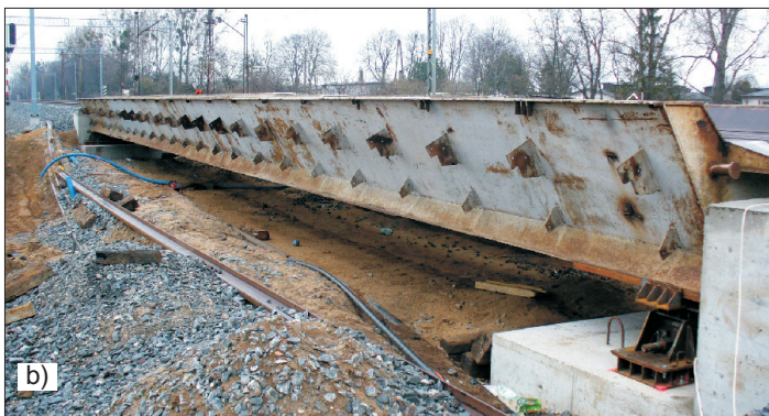
Fig. 1. KO30 bridge span: a) the cross-section scheme, b) the view of the span in service - track No. 2 PKP PLK
