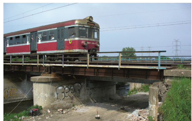
Fig. 4. Field measurements – the bridge under EN57 train
