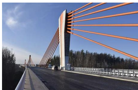
Fig. 1. View of the bridge [15]
