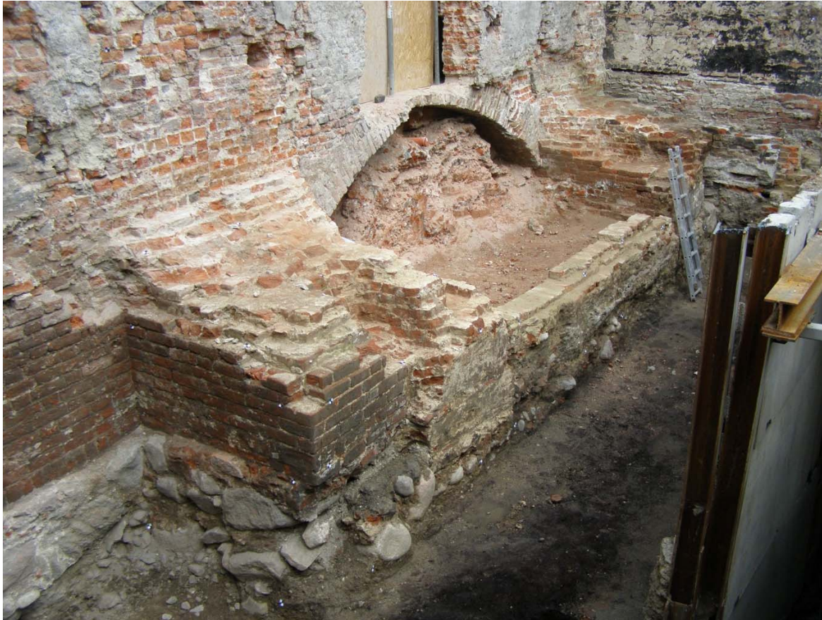
Figure 2. A top view of relics of brick architecture, a fragment of a medieval tower under the Old Pharmacy (source: material made available by the architect Wojciech Narloch)
