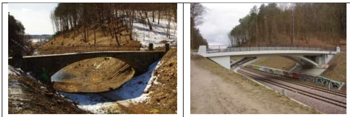
3. Demolished viaduct name of David Weiser (left) and newly built footbridge in the area of street Gomółki in Gdansk Wrzeszcz (photo by Pawel Dabrowski)
