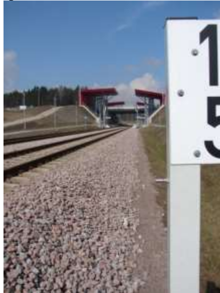
2. Sign of axis adjustment of the track Pomeranian Metropolitan Railway (photo by Pawel Dabrowski)
