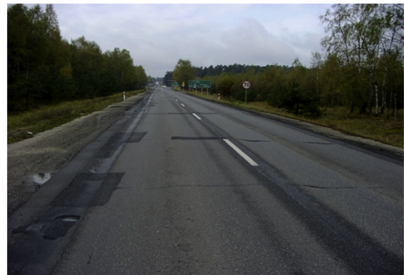
Fig. 1 – Example of a national road pavement qualified for cold recycling.
