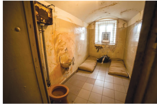
Fig. 4. Former prison in Warsaw – a former cell which belongs to the museum exposition [24]
