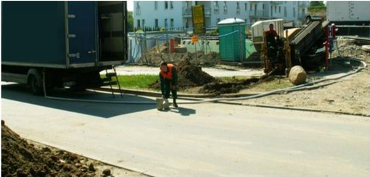
Figure 7. Execution of pilot drilling
