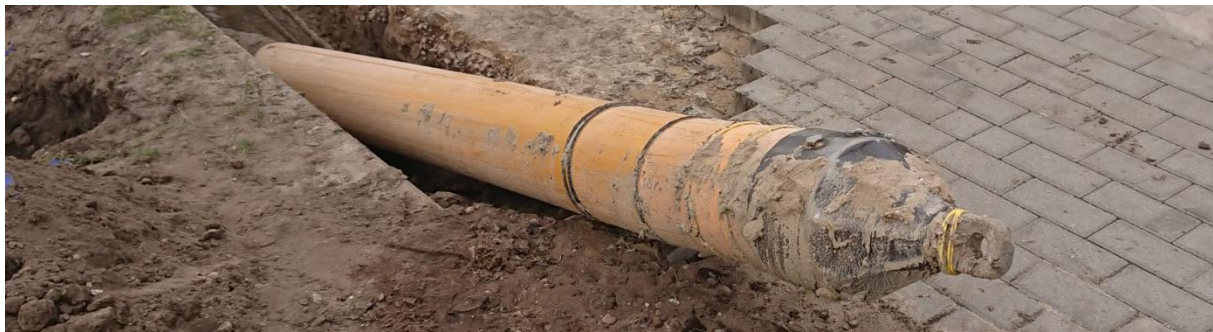
Figure 14. Leading the pipe in the entrance chamber
