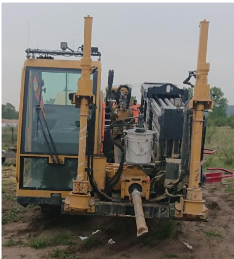
Figure 5. Drilling rig front view.
