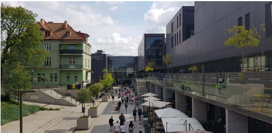
Figure 5. General view of the new Sopot Railway Station complex (2018).
