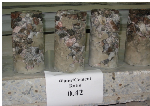
Figure 4. The grout was not able to fill all the voids between coarse aggregates.
