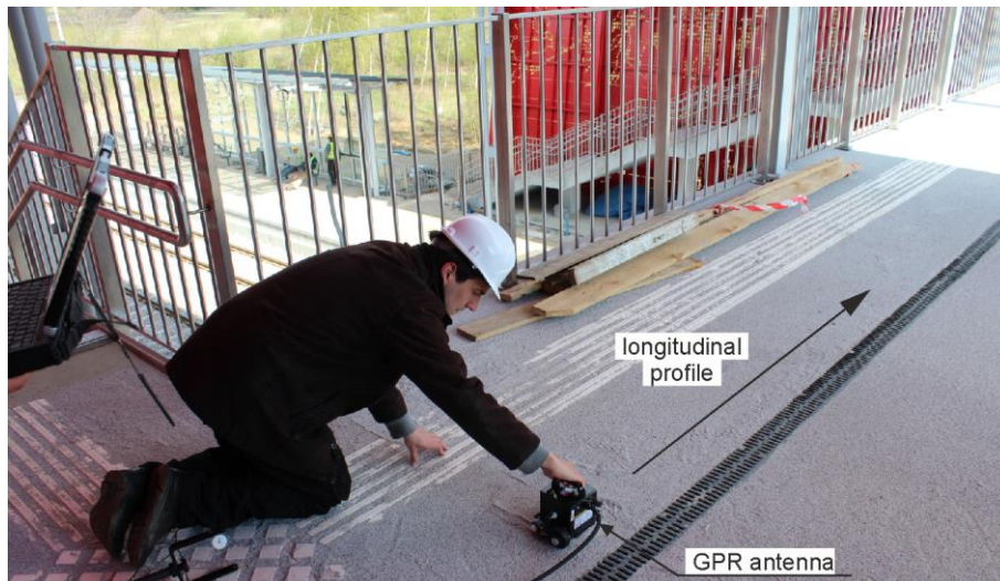
Figure 15. Bridge deck during GPR measurements (Survey #2)
