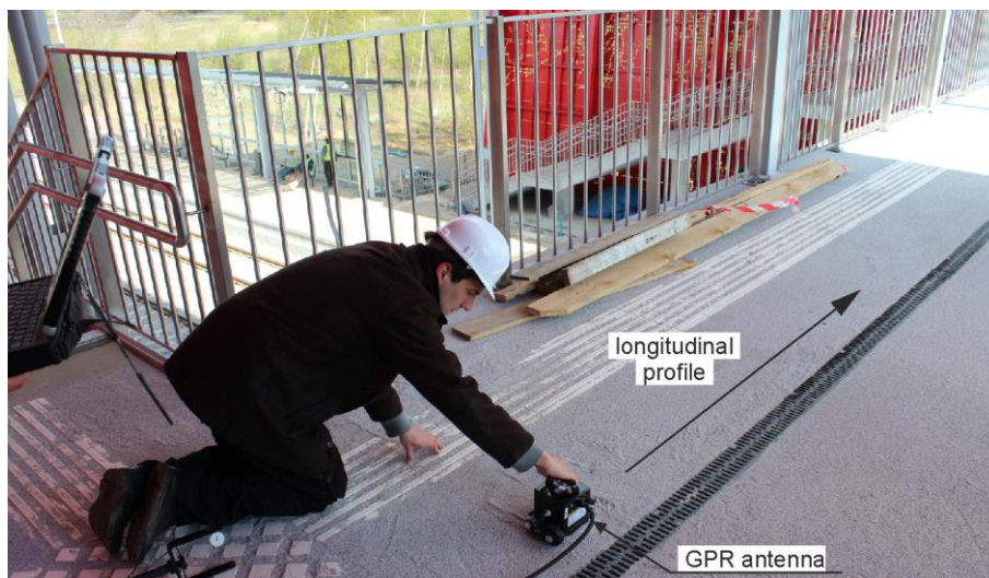
Figure 15. Bridge deck during GPR measurements (Survey #2)
