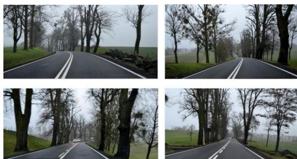
Fig. 9. Identification of hazards on section of NR road 55
