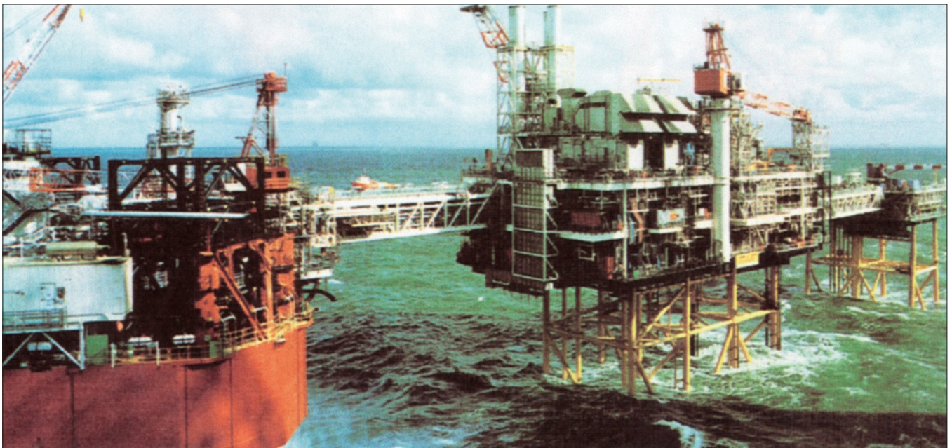
Fig. 5. Offshore platforms with connecting bridges [10]
