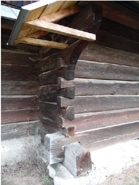
Figure 10. Current condition of log walls with dovetail notches in Chotylub: cracks in log walls in and contemporary repairs of the eaves roof.
