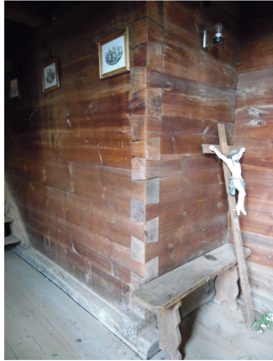
Figure 9. Current condition of log walls with dovetail notches in Chotylub outside and inside.
