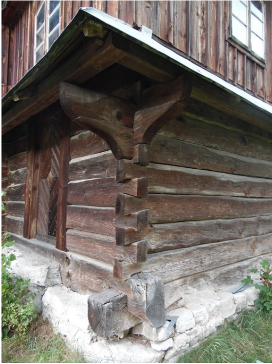
Figure 9. Current condition of log walls with dovetail notches in Chotylub outside and inside.
