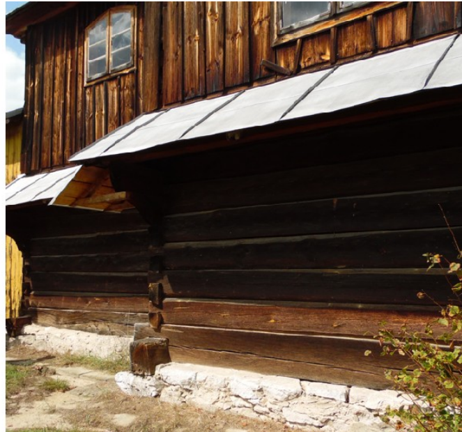
Figure 10. Current condition of log walls with dovetail notches in Chotylub: cracks in log walls in and contemporary repairs of the eaves roof.
