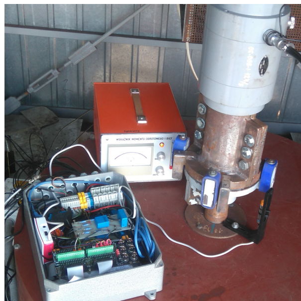
Fig. 2. System for monitoring the operation parameters of a wind farm with a VAWT.
