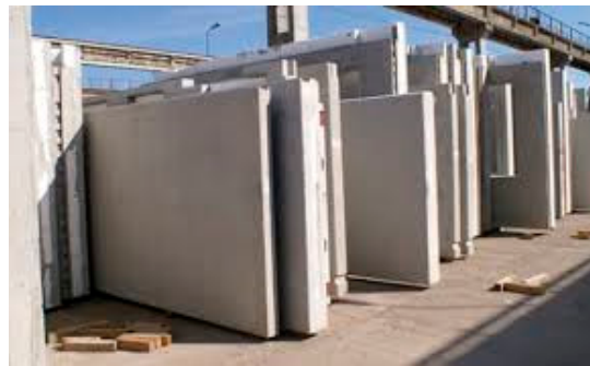
Figure 2. Prefabricated elements storage.
