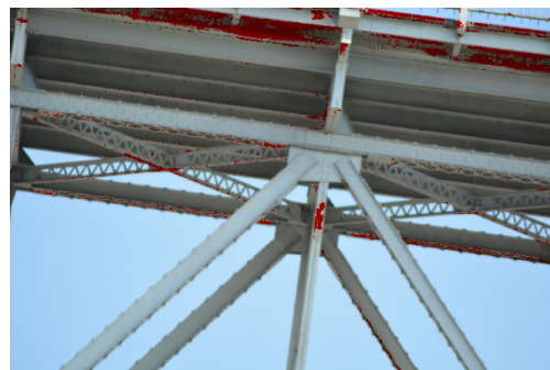
Figure 15. A database of rust colour pixels.
