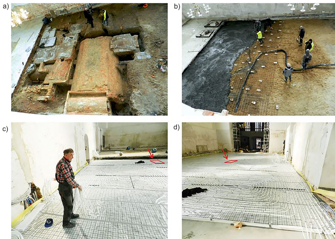
Fig. 1. Photograph of the floor in St. Joseph's Church in Gdańsk, Poland (Google Maps coordinates in a WGS84 system: 54.354111 N, 18.647135 E): a) excavation view, b) concreting of the reinforced concrete slab, c), d) floor heating view with marked locations of the entrances to the crypts.
