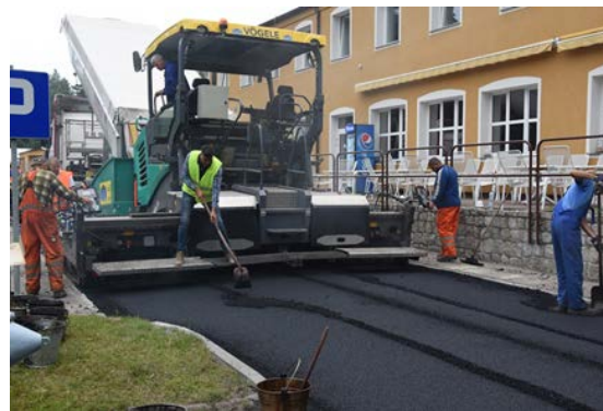
Figure 11. Paving of the poroelastic mixture.
