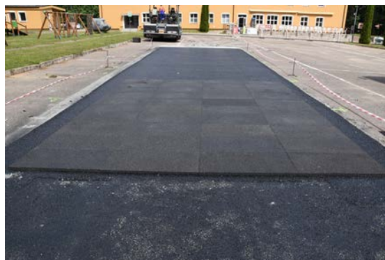
Figure 16. Slabs of Poroelastic Road Surfaces (PERS) polyurethane poroelastic mixture after installation.
