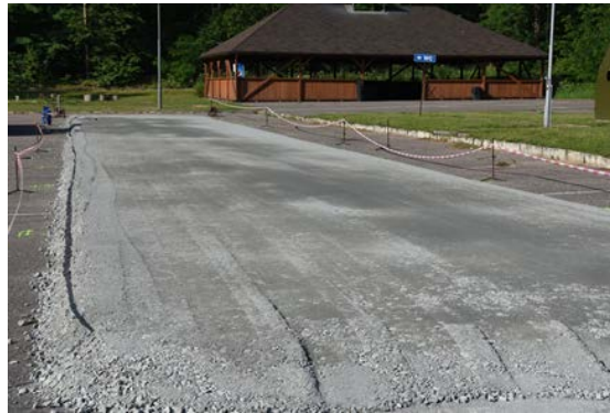
Figure 13. Parking lot area leveled out with the unbound aggregate base course.
