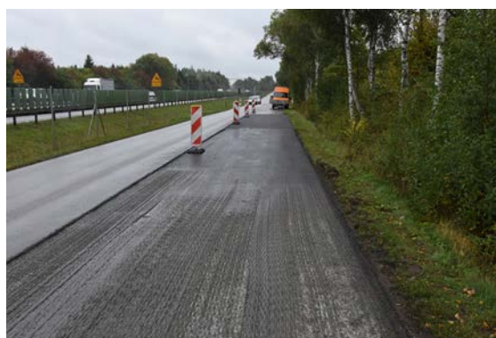
Figure 17. New binder course after surface milling.
