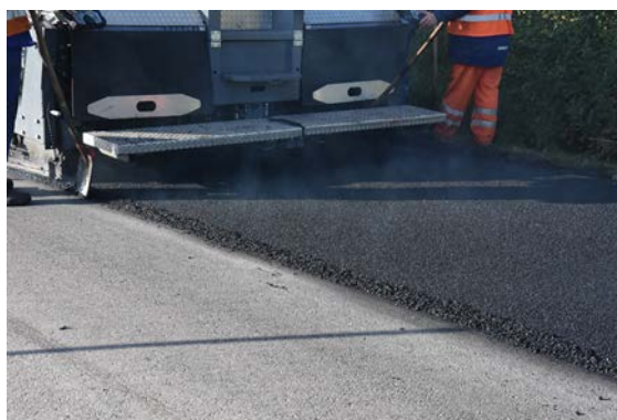
Figure 18. Laying of the poroelastic mixture.
