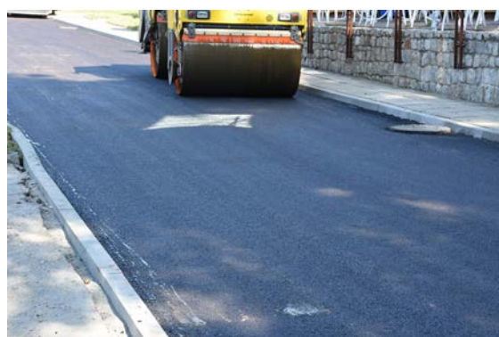
Figure 8. Compaction of the binder course AC 16W.
