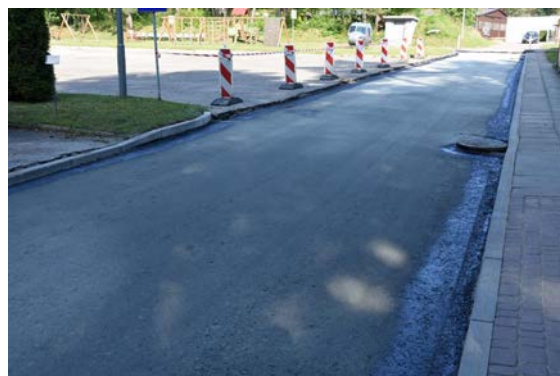
Figure 7. Unbound aggregate base course ready for laying the binder course made of AC 16W.
