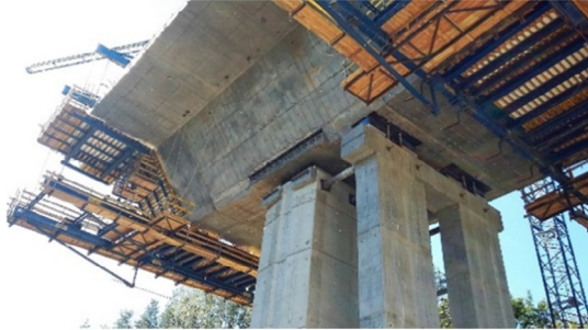
Fig. 10. Monitored section no. 4.4.
