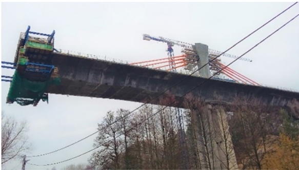
Fig. 11. Monitored section no. 3.18.
