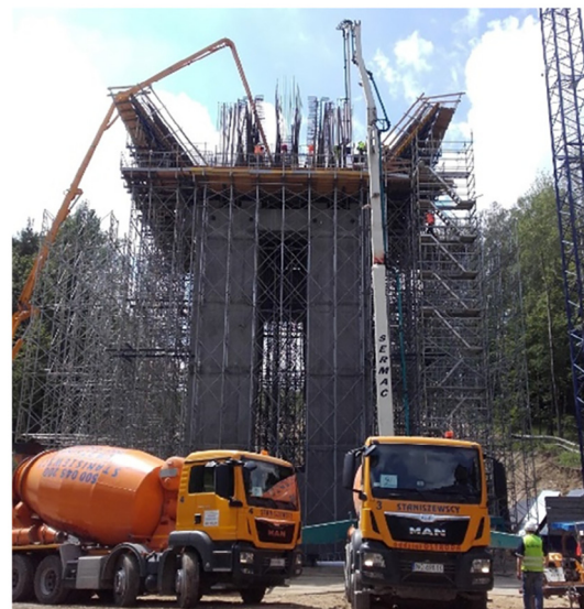
Fig. 9. Monitored section no. 4.1–2.
