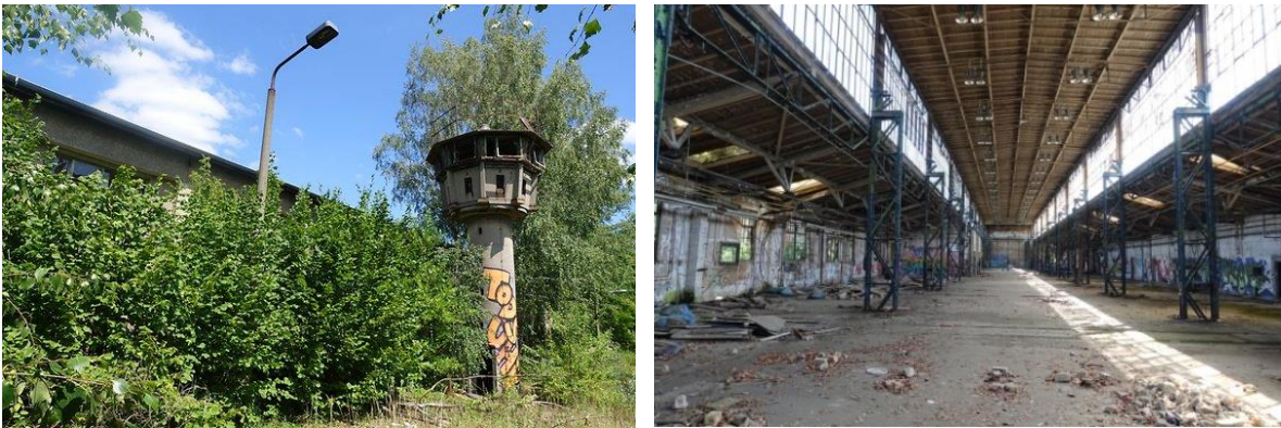
Fig. 14. Dilapidated buildings at the former Johannisthal Airport. Source: (Berliner Zeitung, 2019).
