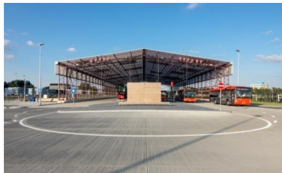
Fig. 12. The hangar in daylight – visible white roof panels. Source: (De architect, 2015).
