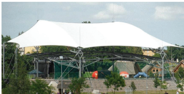
Fig. 1. Membrane hanging roof in Pruszcz Gdanski
