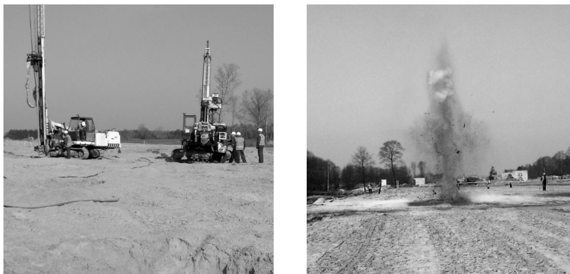
Figure 6. Blasting charge in practice.
