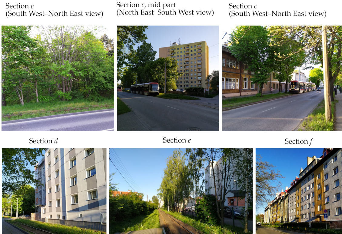
Figure 3. View of the tramway track in the area of sections c , d , e and f .
