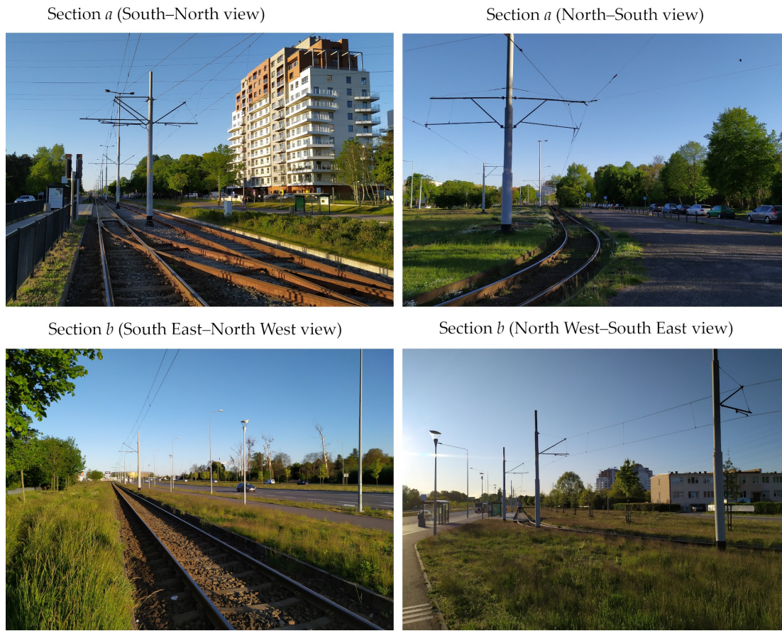
Figure 2. View of the streetcar track in the area of sections a and b .
