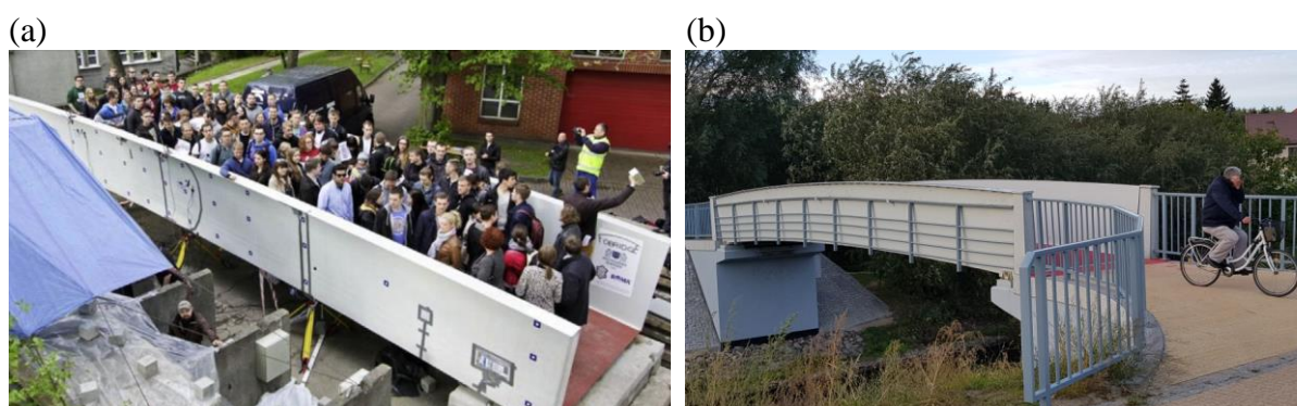
Fig. 1. The footbridge (a) during examination in Gdansk University of Technology campus [46], (b) installed for public traffic over Radunia River near Gdańsk, Poland
