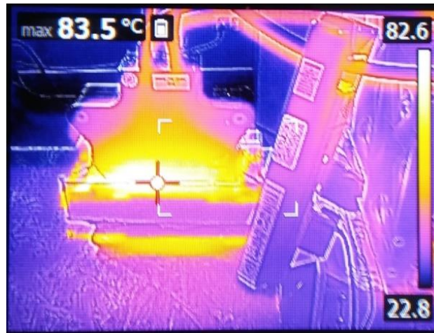
Figure 11. Temperature measurement of the second developed MFT with split windings at power of 45 kW without forced cooling.
