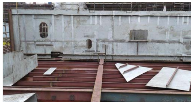
Fig. 1. RSW cargo tank under construction in shipyard
