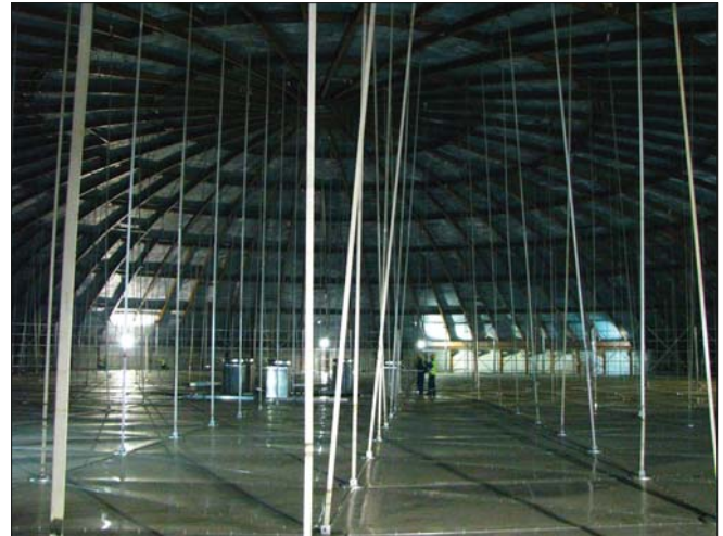
Fig. 3. Underside of the dome and the lightweight inner aluminium roof
