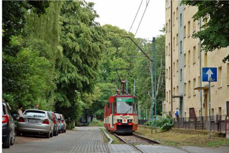
5. The condition of the track and obstacles along the section d
