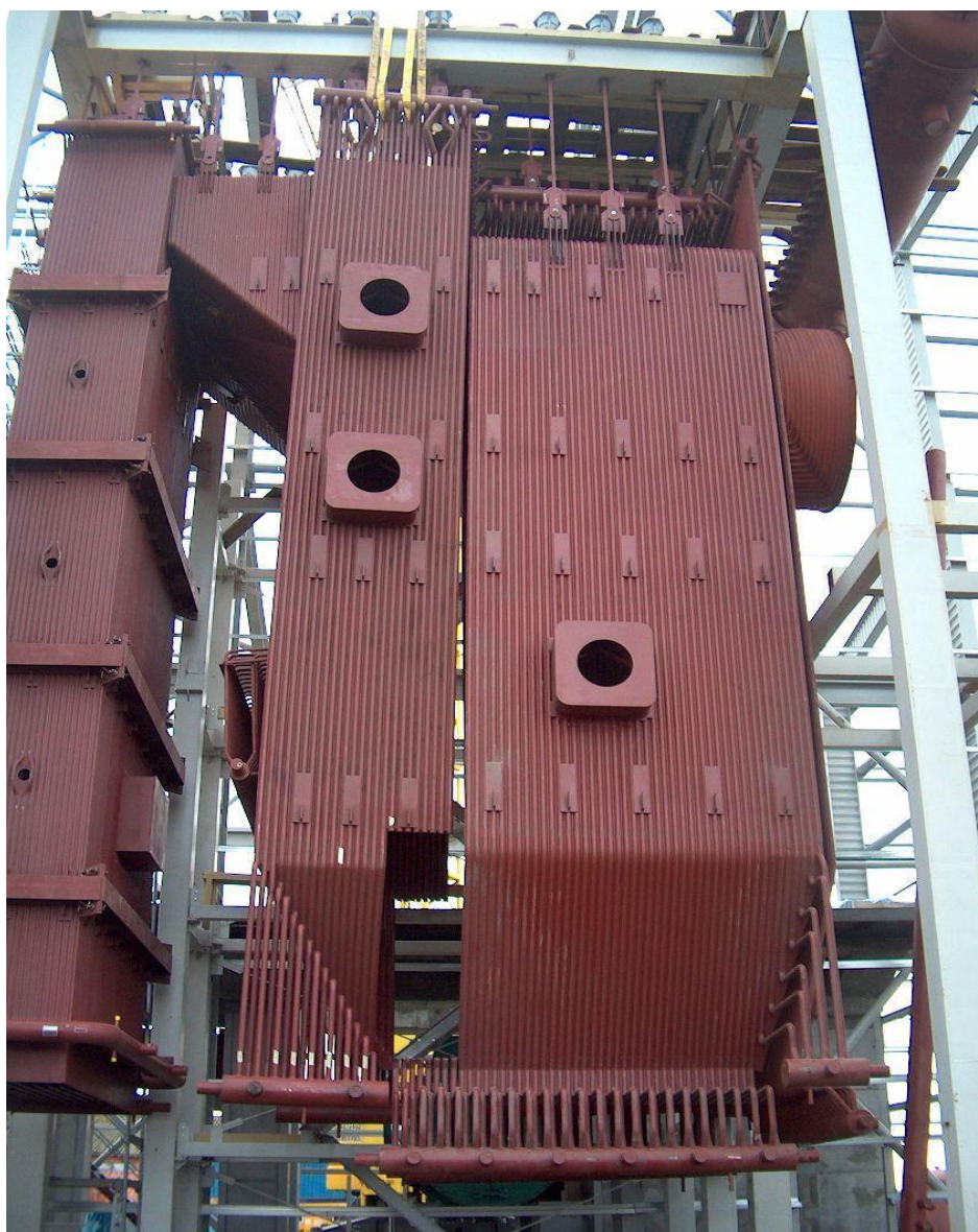
Fig. 4. Fluidized bed chamber.
