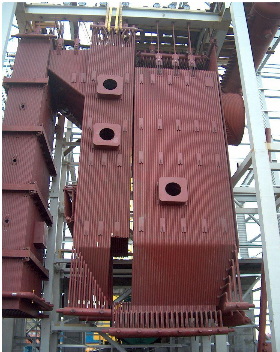
Fig. 4. Fluidized bed chamber.
