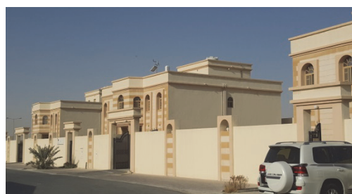
Figure 9. Temporary QNL offices in villas.
