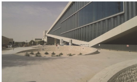
Figure 6. External facade of the QNL building (photo by K. Dudek, Dec 2015).
