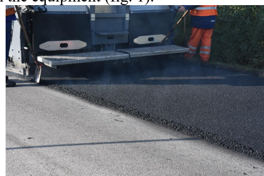
Figure 1. Paving of poroelastic mixture PSMA 5 with highly modified bitumen 45/80-80
