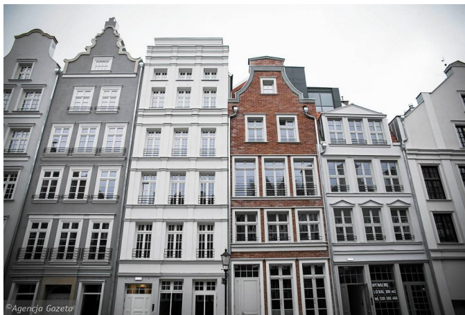
Figure 11. Tenement houses in Św. The Church of the Holy Spirit in Gdańsk; designed by P. W. Kowalski [53].
