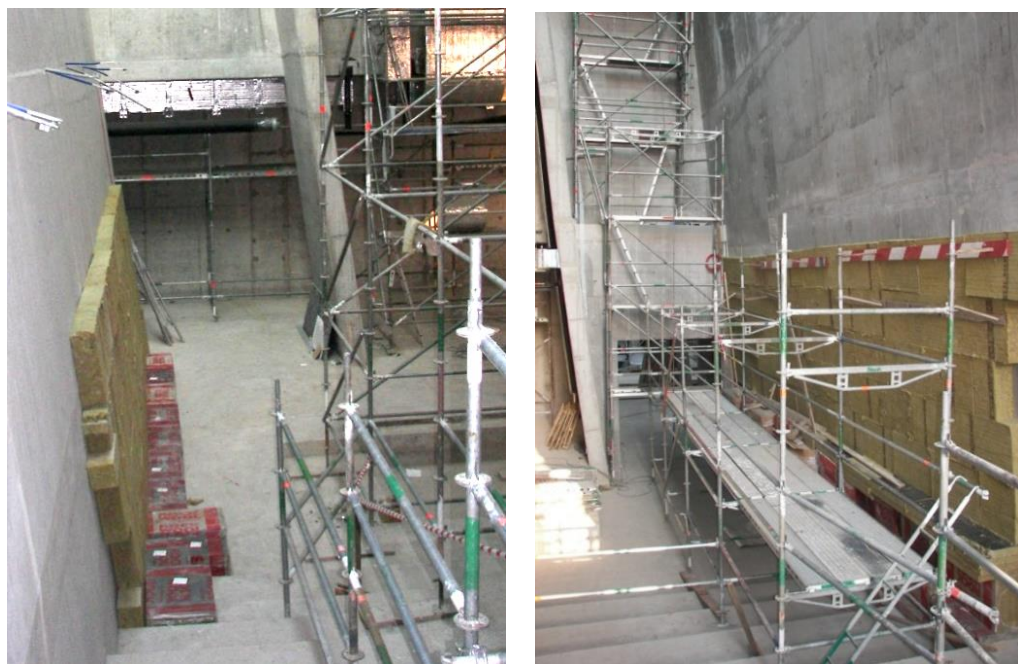
Figure 10. The multi-purpose hall during the acoustic experiment regarding the susceptibility of the room to the formation of the flutter echo. View from the audience on the stage, the left- and right-side walls are shown (photo by A. Kulowski).
