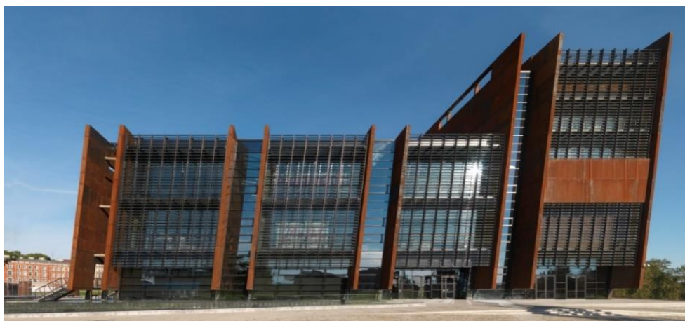
Figure 3. The south and west façade of the ECS, with structural walls which deviate from the vertical by 6.5^\circ . The façades of the ECS are covered with 5 mm thick corten plates (photo by Wojciech Kryński).
