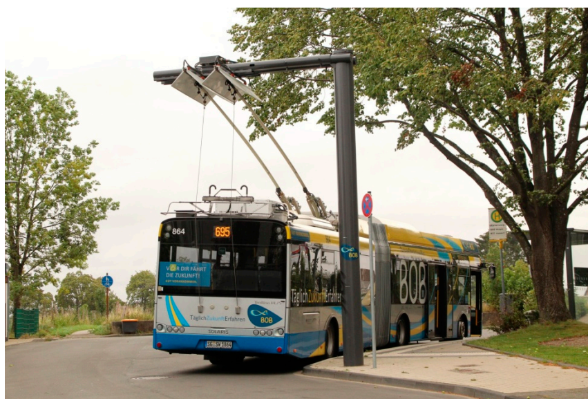
Figure 1. Trolleybus charging station in Solingen (photo taken by M. Bartłomiejczyk).
