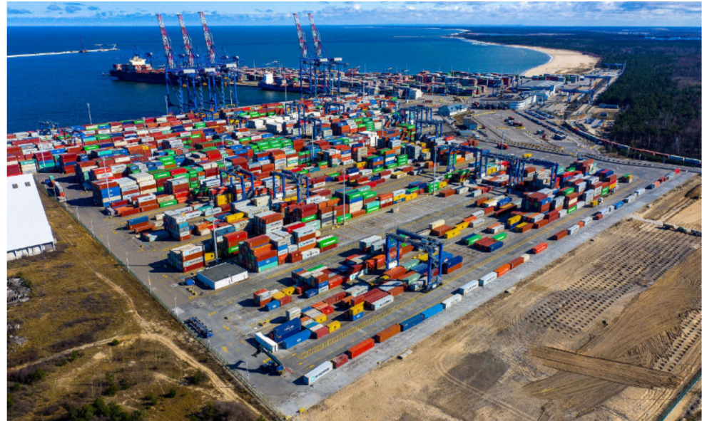
Figure 1. Terminal area—DCT Gdańsk SA.
