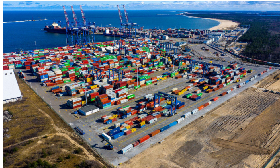
Figure 1. Terminal area—DCT Gdańsk SA.
