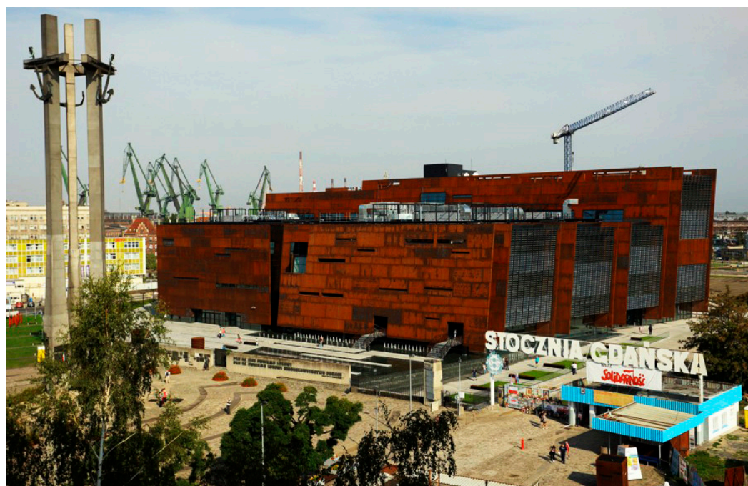
Figure 10. Building of the European Solidarity Centre together with its context: Gate No. 2 (bottom right) and the Monument to the Fallen Shipyard Workers of 1970 (left). Source: Grzegorz Mehring/ECS archive.
