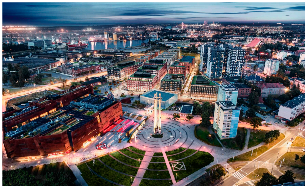
Figure 13. The construction of the DOKI investment became possible after the demolition of some barracks. The project scale is large. The new development is going to infill the area between the ECS (bottom left), the Bastion Wałowa (very densely erected four towers on the upper right—
