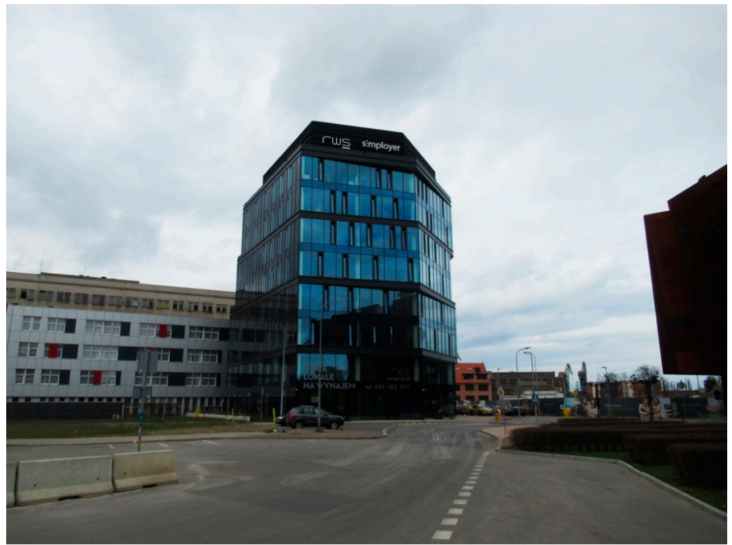
Figure 14. Eternum offices has been constructed just nearby the European Solidarity Centre (the part of the building on the right). It is important to notice the contrast between the new building and the old buildings from the 1970s (on the left) that housed a workers' hotel. Source: authors' archive.
