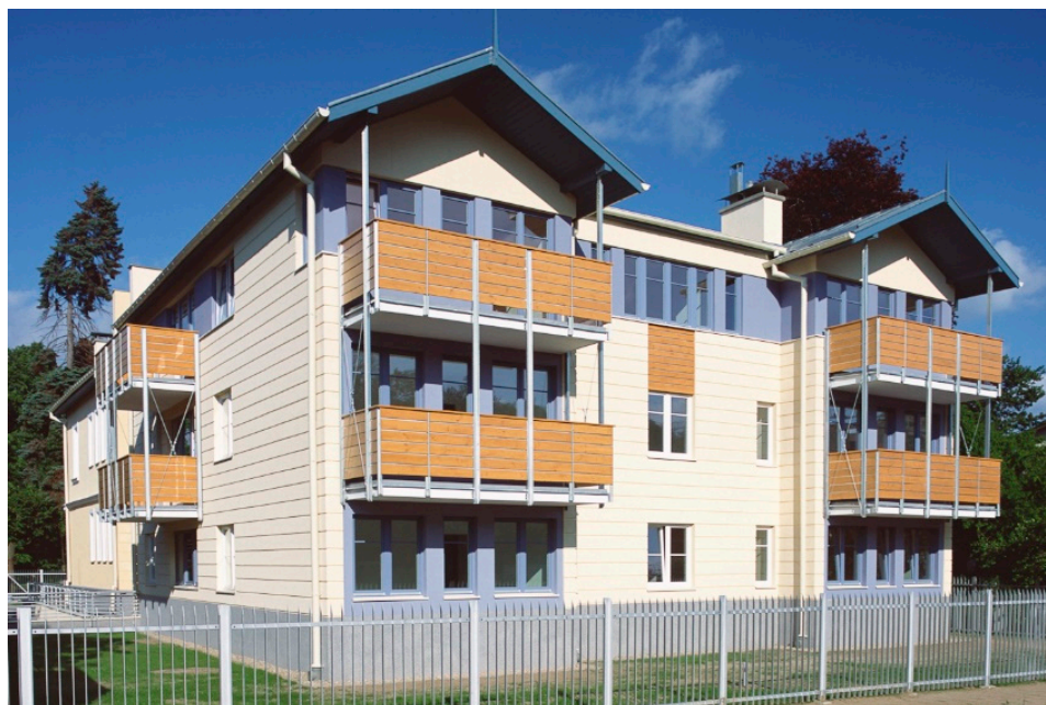
Figure 14. Extended part of Willa Halina. Source: FORT Taraszkiewicz Architekci.
