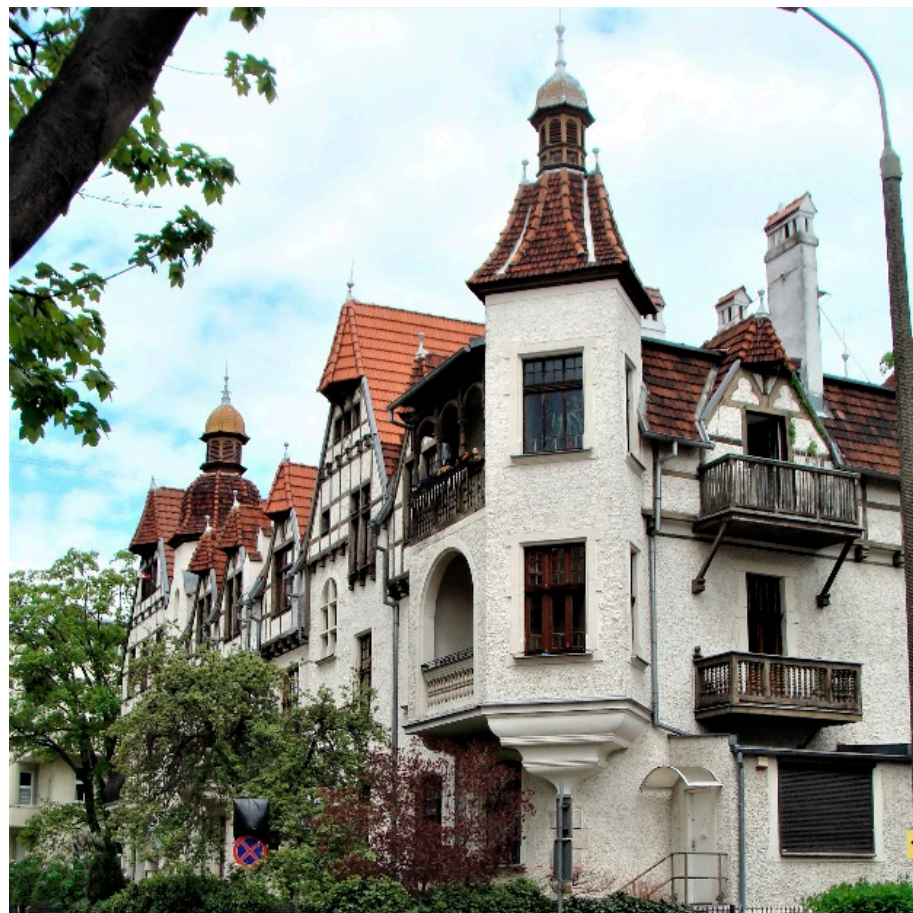
Figure 2. Tenement house from 1905 in Sopot. Source: A. Taraszkiewicz.
