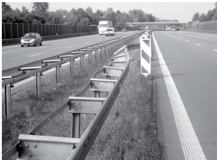
Fig. 1. View of damaged road barrier as a result of vehicle impact, impact angle was approx. 8 degrees (source: GDDKiA)
