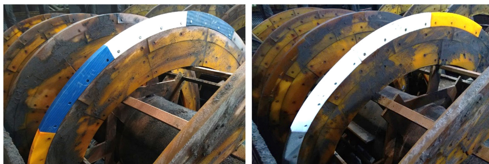
Figure 6. View of the installed test linings—before starting the test.
