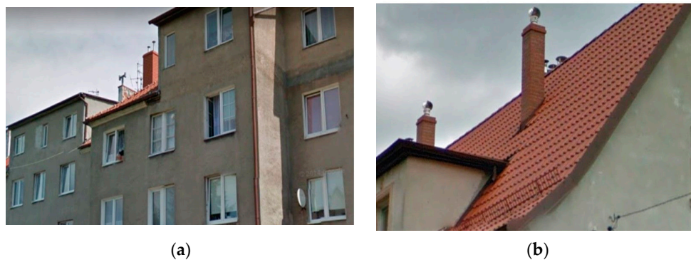
Figure 21. Multi-family housing in Gdańsk: (a) traditional chimney cap and (b) rotary type chimney cap.
