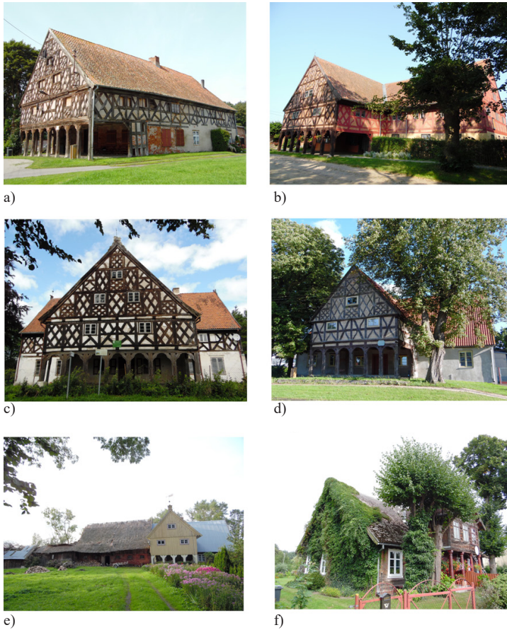
Fig. 1. Types of arcaded houses: a) type I house in Klecie, b) type II house in Trutnowy, c) type II-III house in Stalewo no.14, d) type III house in Koszwały, e) type III house in Markusy, f) type III house in Mikoszewo no. 68 (photo by the author)
