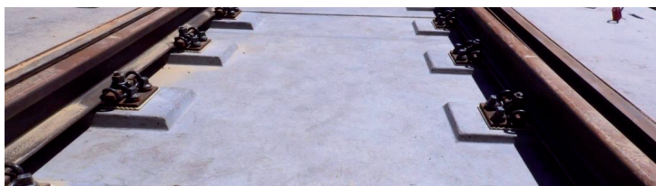
Fig. 7. Module of the level crossing during construction
