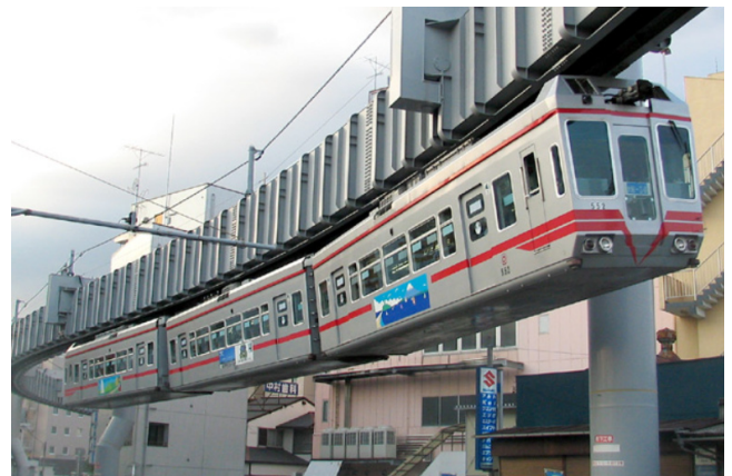
Fig. 3. Vehicle on Shonan Monorail line [8] Rys. 3. Pojazd na linii Shonan Monorail [8]
