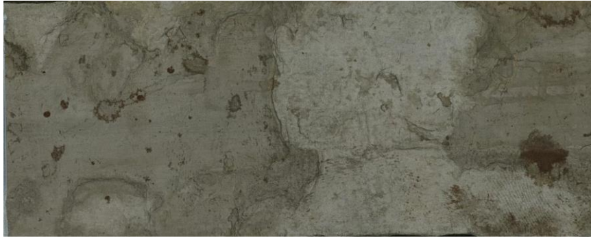
Figure 4.17. An example of a scan of the corroded surface (specimen 6.3).
