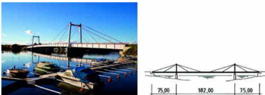
Fig. 13. Strömsund Bridge, Sweden, 1956 [5] (photo: wikipedia.com)
