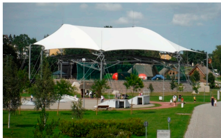
Figure 1. Membrane hanging roof co-designed by the authors in Pruszcz Gdanski, Poland.
