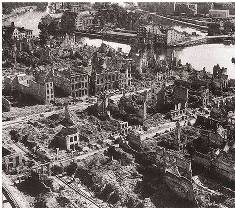
Figure 1. Photograph of damage in Gdańsk after the Second World War. Source: (Cieślak and Biernat 1994)
