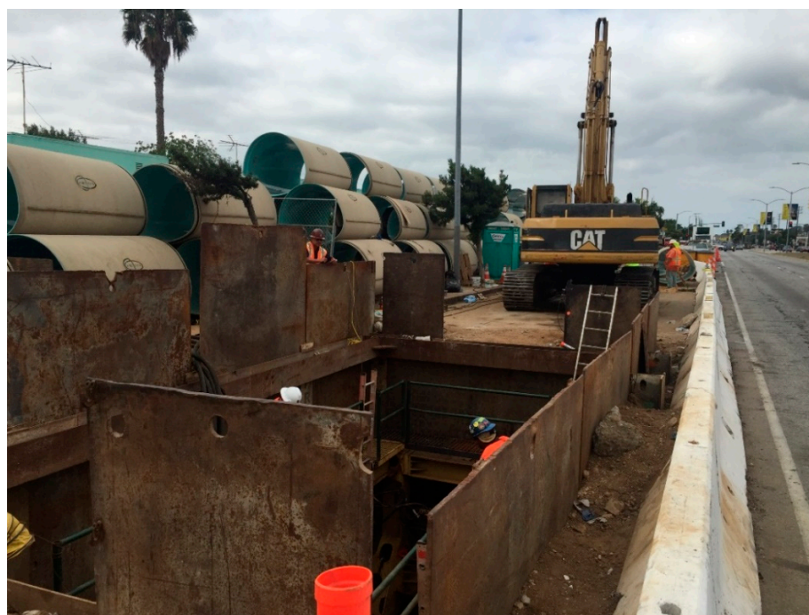
Figure 16. Installation access pit with stored segments of non-circular pipeline [34].
