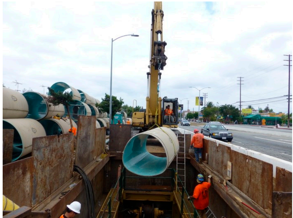
Figure 17. Lowering the segment into the pit [34].
