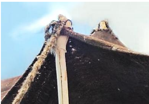
Fig. 117:Garapapakh Tribe. The columns are forked at the top and the end one has a roof cover loop and a stretching rope attached, photo by author
