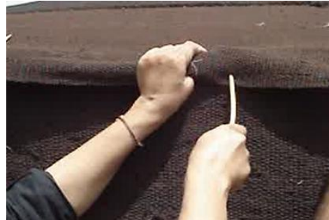
Fig. 86: Piercing the cover with thin pins in roughly 20 cm distances to brace the edge, photo by author
