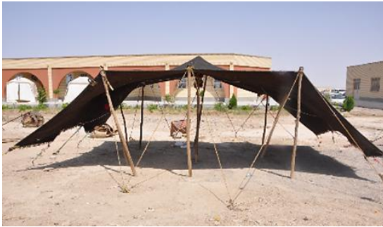
Fig. 122: Bahlooli Tribe. View of a Black Tent cover and position of its columns, photo by author
