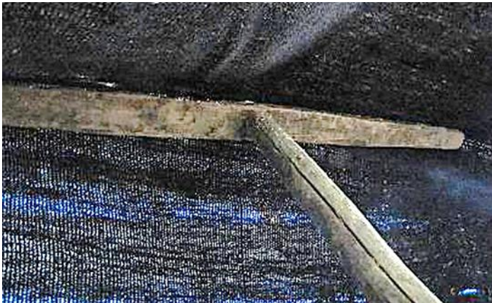
Fig. 115:YaromTatli Tribe.The central column of the tent and its pass from the carrier beam on it to slope the tent, photo by author
