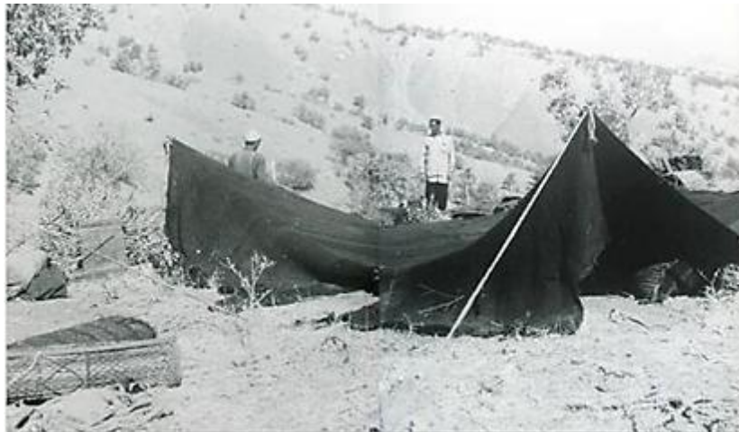
Fig. 78: Corner posts on both sides are lifted, photo by, Edelberg.1964, source: Digard, J.P., 1990, p. 117
