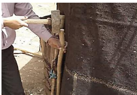
Fig. 87: Thin branches are rammed/pounded into the ground and Chigh is unwind to support the wall, photo by author
