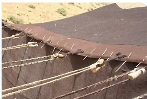
Fig. 85: Wall and roof of the tent are connected by wooden pins, photo by author
