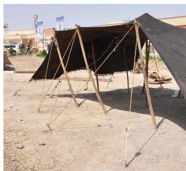
Fig. 121: Bahlooli Tribe. Zig-zag rope joins pins and columns around the tent, photo by author
