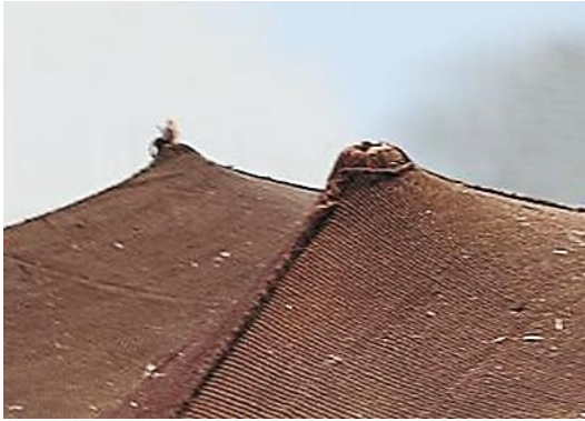
Fig. 119:Kormanj Tribe, the openings in the fabric where the tips of columns stick out protected from inside and outside from water leakage, photo by author
