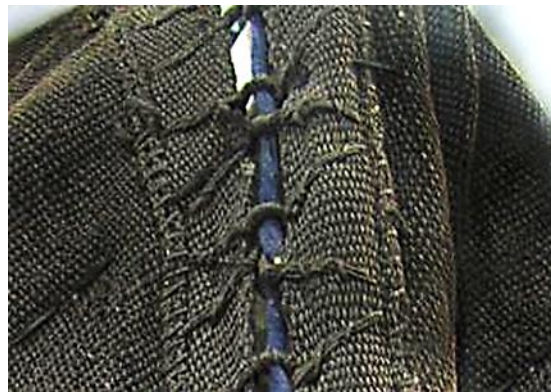
Fig. 114:YaromTatli Tribe. Method of connecting two sheets on the ridge of the roof. Two upper-most strips of fabric have sewn-on loops on their edge. The rope which is threaded through those loops joins the parts of the roof, photo by author
