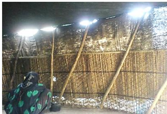
Fig. 111: Columns around of the tent, photo by M. Moghadam
