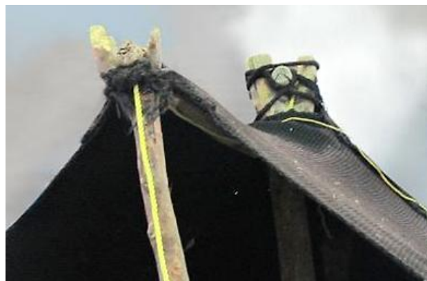
Fig. 127: Soleimani Tribe. columns with a groove/forked end and placement of horizontal beams on them, photo by author
