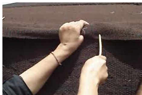
Fig. 86: Piercing the cover with thin pins in roughly 20 cm distances to brace the edge, photo by author
